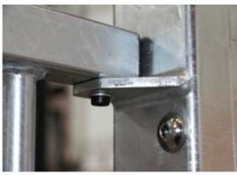
All steel components are manufactured from carbon steel, welding's according EN ISO 5817 & Hot dip galvanised (HDG) according to ISO1461. This process ensures good protection in all circumstances.
