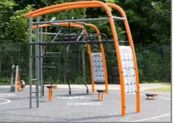
For ensuring the integrity of the main frame, the orange coloured main posts are made of ø101.6 x 3mm steel posts, which are hot dip galvanised and powder coated Orange (RAL2010). The supportive posts receive the same surface treatment and are made of ø76.1 x 3.6mm steel tubes, powder coated grey (RAL7012).
