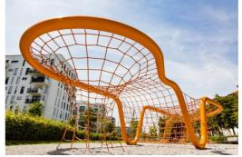
The steel surface of these bended steel pipes are wet painted with one basic layer and one top layer of lead free colour material. The paint has excellent corrosion resistance and can be easily maintained.
