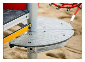
Grey round post decks are supported by hot dipped galvanized steel and made of molded 75% post-consumer PP material with a non-skid pattern and texture surface.
