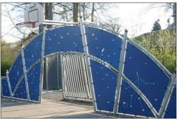
The goal measures ~140cm in depth and ~330cm in width with all posts made of galvanized steel with a hot dip galvanized surface treatment. The front frame is made with Ø48 tubing, and the backside of the goal uses 10 tubes with a diameter of ø38.
