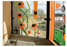
Panels are manufactured from high-quality polycarbonate with a thickness of 15mm. The graphic prints are added by a unique multi-layer print process where the inner layer is the image and outer transparent layer functions as protection. Both PC panel and the water-based lacquer are UV stabilised to prevent fading.
