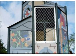
Fully welded steel frame with 45° cross welded steel grid of round steel pins with a diameter of 4mm. The airflow panel contributes to the overall structural integrity of the GIANT towers.
