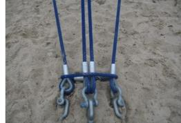
The huge spacenet structures are secured to the foundation with a system of three turnbuckles. Horizontal and vertical edge cables are fixed to individual turnbuckels, which then connect to individual steel anchors. This system ensures that each edge cable can be tensioned separately and increases structural safety by way of independent anchoring.
