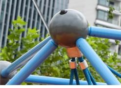
The metal parts are made of high quality steel, hot dip galvanized inside and outside with leadfree zinc. On the outside, there is an additional layer of powder coating. This ensures both excellent corrosion resistance and colorful design expression.
