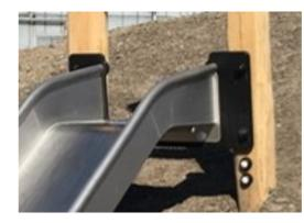
Slide interface panel of 19mm EcoCore<sup>™</sup>. EcoCore<sup>™</sup> is a highly durable, eco-friendly material, which is not only recyclable after use, but is also made of +95% recycled postconsumer material from e.g., food packing waste in both core and colorful outer layer.
