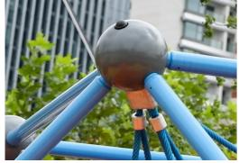
The metal parts are made from high-quality steel consisting of hot-dip galvanisation on both the inside and outside and also includes leadfree zinc and an additional layer of powder coating. This ensures both excellent corrosion resistance and colourful design expression.
