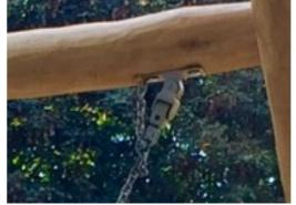
Swing hangers for Robinia wood crossbeams are made of stainless steel brackets and can move over two axes. The flange bearings are silicone enriched to make the suspension maintenance free.
