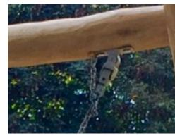
Swing hangers for Robinia wood crossbeams are made of stainless steel brackets and can move over two axes. The flange bearings are silicone enriched to make the suspension maintenance free.
