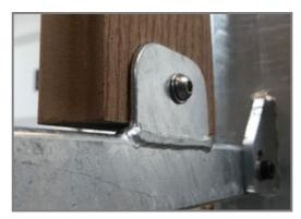
The WPC boards are attached to 70 x 45 x 3mm welded flanges with stainless steel M8 bolts, nuts and washers. These connections are not visible from the inside and create a safe and robust connection.
