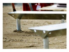
The cubes are supported by a unique designed footing system that secures the correct positioning of the cubes.
