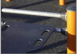
The surface is made of Ekogrip<sup>™</sup> panels, consisting of 15mm polyethylene with a 3mm top-layer of thermoplastic rubber. The Ekogrip™ panels have a non-skid effect for comfortable and safe training at all weather circumstances.
