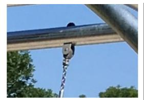
Unique designed swing hangers of stainless steel with anti-twist function. The hangers are attached to the cross beam by a bolt through connection to ensure high durability.
