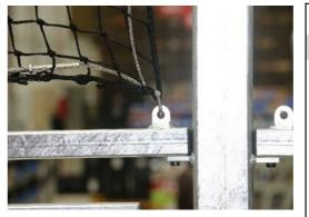
The net is made of a Ø4mm black polypropylene, better known as Nylon, with a mesh size of 45 x 45mm and reaches till 5m high. The nets will keep all balls in the MUGA and retains the transparency.
