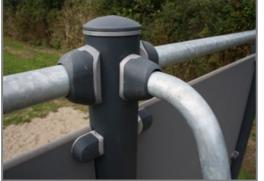
The connectors are made of die-cast aluminium, specially alloyed for the outdoor environments and heavy usage. The screws attaching the connectors are stainless steel and protected by zinc washers.
