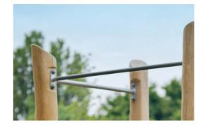
The pull up bar is made from  $\ensuremath{\emptyset32}$  mm HDG steel bar. The bar is 1080mm wide and 2300mm above ground
