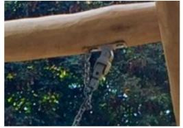
Swing hangers for Robinia wood crossbeams are made of stainless steel brackets and can move over two axis. The flange bearings are silicone enriched to make the suspension maintenance free.
