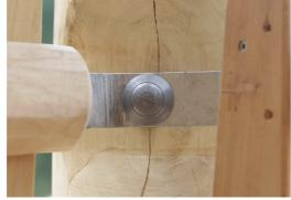
The hardware is made of stainless steel or galvanised steel to ensure durable connections that has high corrosion resistance.
