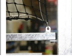
The net is made of a Ø4mm black polypropylene, better known as Nylon, with a mesh size of  $45 \times 45$ mm and reaches till 5m high. The nets will keep all balls in the MUGA and retains the transparency.
