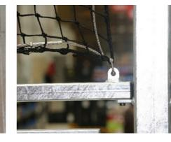
The net is made of a Ø4mm black polypropylene, better known as Nylon, with a mesh size of 45 x 45mm and reaches till 5m high. The nets will keep all balls in the MUGA and retains the transparency.a
