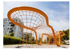
The steel surface of these bended steel pipes are wet painted with one basic layer and one top layer of lead free colour material. The paint has excellent corrosion resistance and can be easily maintained.
