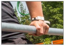
The bars intended for exercises are made of hot-dip galvanised steel ø48mm. The diameter of these bars provide a good support when used to for push ups exercises or when doing exercises standing on the tubes.
