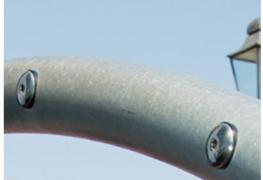
The steel structures are hot-dip galvanised inside and outside with lead free zinc. The galvanisation has excellent corrosion resistance and requires low maintenance.
