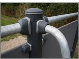
The connectors are made of die-cast aluminium.
